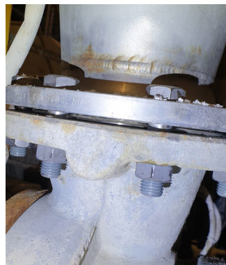
AFTER INSTALLATION OF DELTAV-SEAL™
