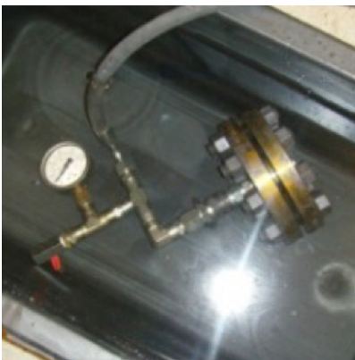
Figure 12. Helium testing - 5 barg
