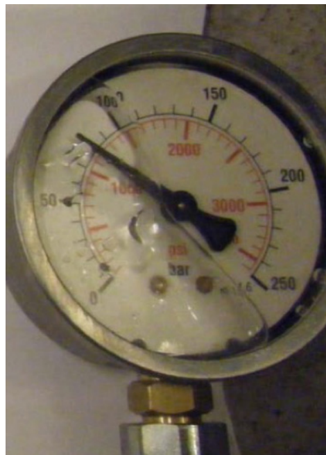
Figure 20. Water testing - 78 barg
