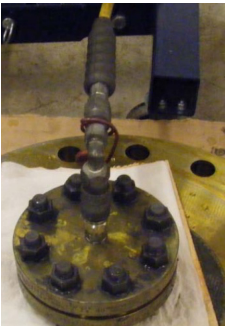
Figure 19. Water testing - 78 barg
